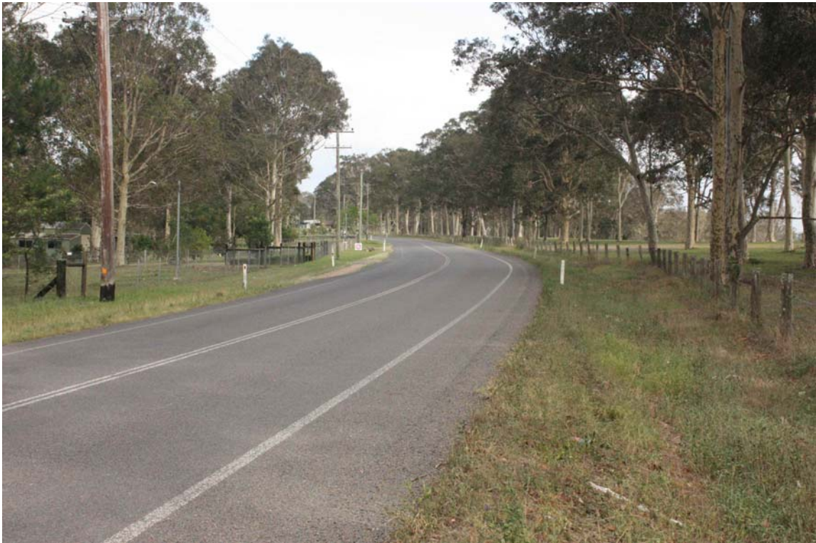
Photo No. 3: Looking right (generally north) along Seaham Road from the showing the existing traffic environment and available sight distance.
