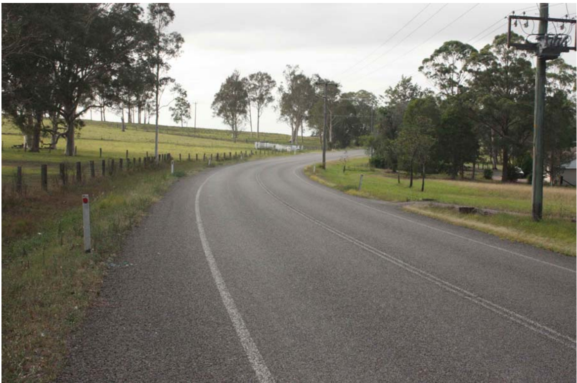
Photo No. 2: Looking left (generally south) along Seaham Road from the showing the existing traffic environment and available sight distance.
